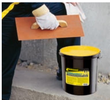
Using a spatula, Gumoasfalt SA 27 is applied on a vertical wall.
