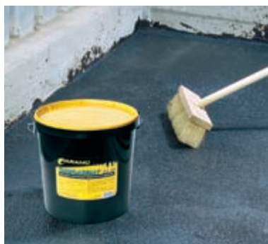
Gumoasfalt SA 12 coat is applied on primed concrete using mop or brush.
