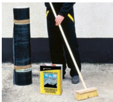
Prior to laying waterproofing felt, the surface needs to be carefully cleaned.
