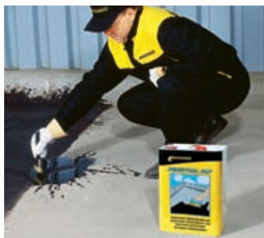
Priming of concrete using PENETRAL ALP paint.
