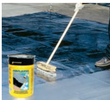
Applying final coat of aluminum-bitumen paint.
