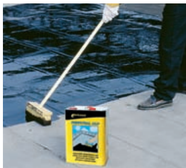
Renewal coat on old roofing using PENETRAL ALP and mop.
