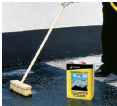
Priming concrete base using a mop.
