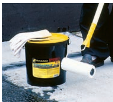
Laying SA 23 on new waterproofing felt, its lifetime is increased and UV protection is upgraded.
