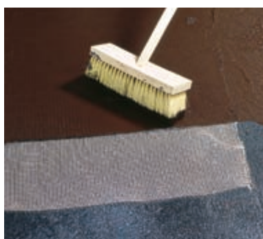
On glass fabric SA 12 is applied using mop or roller.
