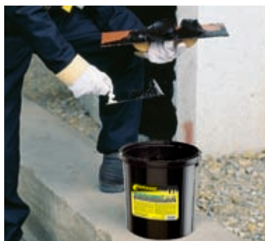
Material is ready for distribution after proper mixing of powder hardener (component B) and bitumen mass (component A).
