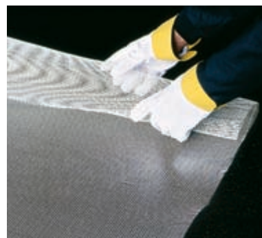
Laying glass fabric on the first layer of SA 12.
