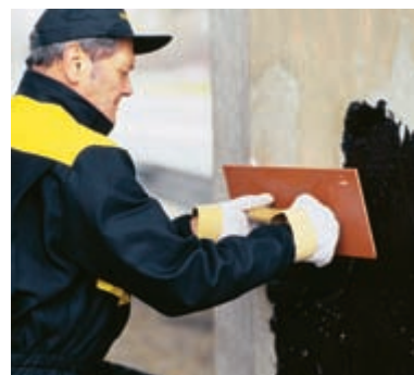
SA 27 is applied from bottom to the top. At least, one layer of 4 mm width must be applied.
